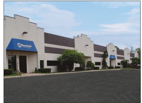
European Sales Office and Warehouse
